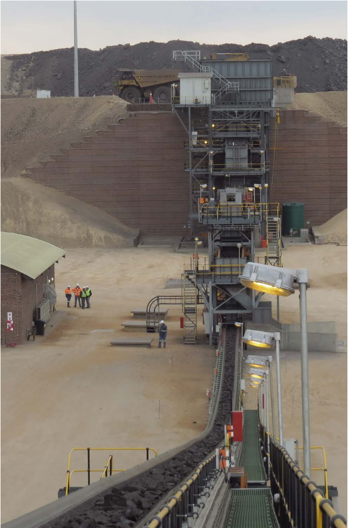
Commissioning of the primary crusher at Tshipi Borwa.
