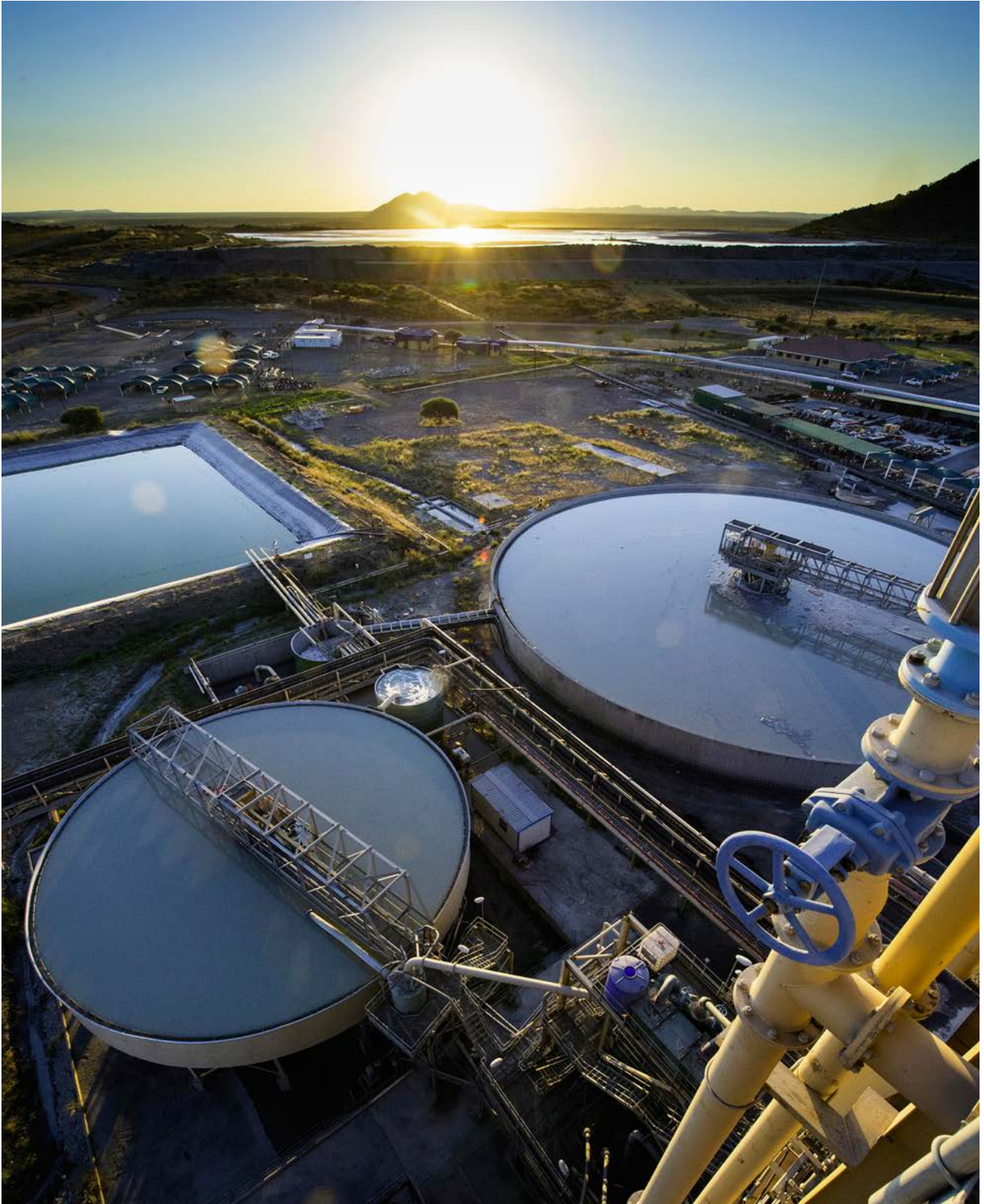
Thickeners and tailings dam at the Pilinghurst Platinum Mine.
